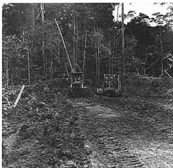
Sappers from 22 Construction Squadron at work on the Keningan-Sepulot road in Sabah. (AWM LES-06/261/MC)
