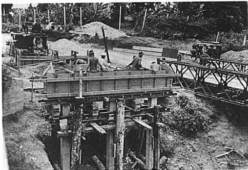
Sappers of 4 Troop, Royal Australian Engineers, 11th Independent Field Squadron, Royal Engineers, constructing a bridge at Lubok Segintah, Malaya, 1955. (AWM P1325/45/12)
